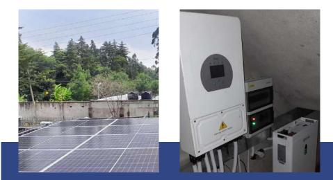
Customer: JEMI GREEN Type: rooftop solar power plant Installed capacity: 6.49 kWp Region: Nyeri county Solar modules: JA Solar 590 W Bifacial Inverters: DEYE 5kw 48v, SUN-5K-SG03LP-EU,single phase Battery:10kwh U-HOME LITHIUM ION BATTERY Year of implementation: 2024 Works performed: design, supply of equipment and materials, installation and commissioning
