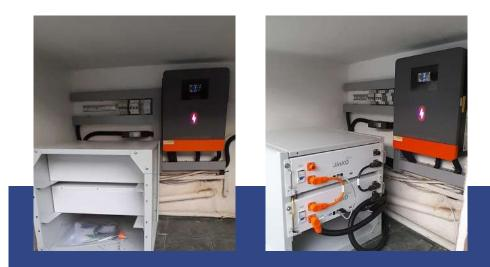
Customer: JEMI GREEN Type: rooftop solar power plant Installed capacity: 6.6 kWp Region: Nairobi county Solar modules: JINKO Solar 600 W Bifacial Inverters: SOLAR INVERTER Battery:10kwh JINKO LITHIUM ION BATTERY Year of implementation: 2024 Works performed: design, installation and commissioning
