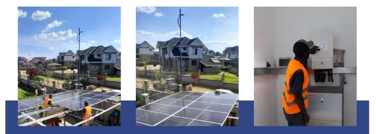
Customer: JEMIGREEN LTD Type: Carpark solar power plant Installed capacity: 7.5 kWp Region: Eldoret, Uasin Gishu county Solar modules: LONGI 625 W Inverters: DEYE 8kw 48v, SUN-8K-SG03LP-EU, single phase Battery:10kwh MEGA TANK GL LITHIUM ION BATTERY Works performed: design, supply of equipment and materials, installation and commissioning
