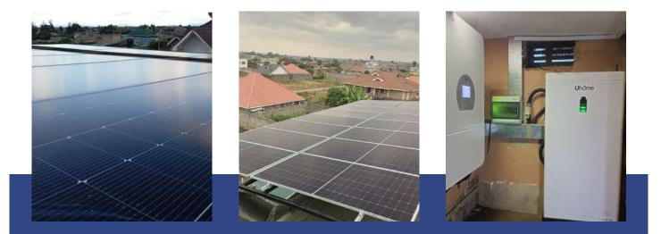
Customer: JEMIGREEN LTD Type: rooftop solar power plant Installed capacity: 10 kWp Region: Ruiru,Kiambu county Solar modules: JINKO 625 W Bifacial Inverters: DEYE 8kw 48v, SUN-8K-SG03LP-EU,single phase Battery:20kwh U-HOME LITHIUM ION BATTERY Works performed: design, supply of equipment and materials, installation and commissioning
