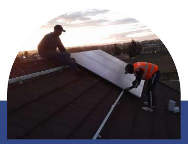
Customer: Mr. Kevin Hela Type: rooftop solar power plant Installed capacity: 4.6 kWp Region: Nairobi county Solar modules: JA Solar 575 W Bifacial Inverters: DEYE 5kw 48v, SUN-5K-SG03LP-EU,single phase Battery:10kwh BYD LITHIUM ION BATTERY Works performed: design, supply of equipment and materials, installation and commissioning
