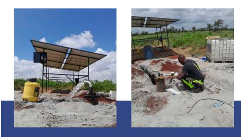
Customer: Mr. MULA Type: shade solar power plant Installed capacity: 6kWp Region: MASIMBA KAJIADO COUNTY Solar modules: LONGI SOLAR 375 W Inverters: 5.5KW VIECHI SUNVERTER, THREE PHASE Works performed: design, installation and commissioning.
