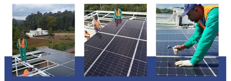
Customer: JEMIGREEN LTD Type: rooftop solar power plant Installed capacity: 12.6 kWp Region: Uasin Gishu county Solar modules: JA Solar 625 W Bifacial Inverters: DEYE 8kw 48v, SUN-8K-SG03LP-EU,single phase Battery:20kwh UHOME LITHIUM ION BATTERY Works performed: design, supply of equipment and materials, installation and commissioning
