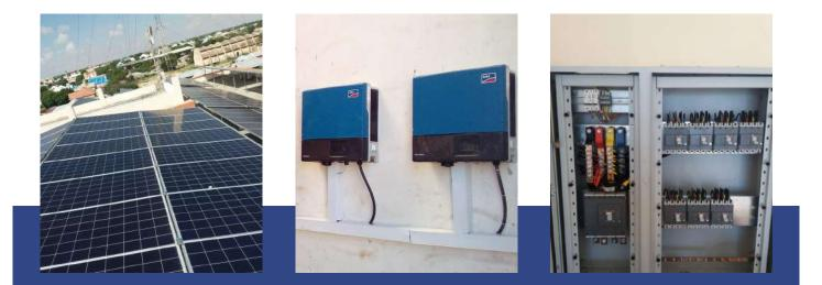
Customer: AUTOMAX ENGINEERING LTD Type: Rooftop solar power plant Installed capacity: 160kWp Region: MOGADISHU SOMALIA Solar modules: AMERI SOLAR 375 W Inverters: SMA 25kw, three phase Works performed: Installation
