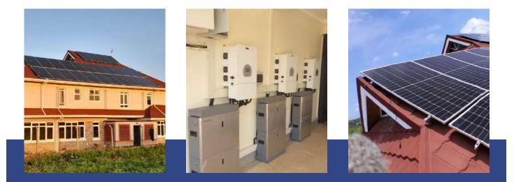
Customer: MADAM CATHERINE Type: Rooftop solar power plant Installed capacity: 24 kWp Region: THIKA GREENS KIAMBU COUNTY Solar modules: JA SOLAR 590W BIFACIAL Inverters: DEYE 8kw 48v, SUN-8K-SG03LP-EU, single phase Battery: 30kwh MEGA TANK GL LITHIUM ION BATTERY Works performed: design, supply of equipment and materials, installation and commissioning
