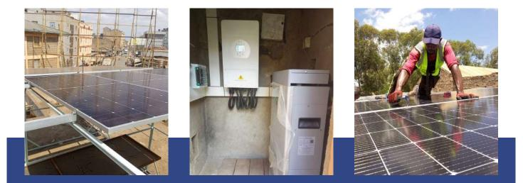
Customer: ALKIN ENTERPRISE LTD Type: Shade solar power plant Installed capacity: 6 kWp Region: Juja,Kiambu county Solar modules: LONGI 600 W Inverters: DEYE 5kw 48v, SUN-5K-SG03LP-EU,single phase Battery:10kwh MEGA TANK GL LITHIUM ION BATTERY Works performed: design, supply of equipment and materials, installation and commissioning
