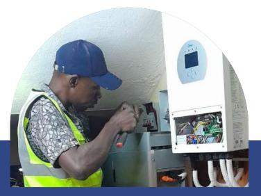
Customer: ENG KIMINGI Type: rooftop solar power plant Installed capacity: 3.6 kWp Region: Juja Kiambu county Solar modules: LONGI 600W Inverters: DEYE 5kw 48v, SUN-5K-SG03LP-EU, single phase Battery:15kwh MEGA TANK GL LITHIUM ION BATTERY Works performed: design, supply of equipment and materials, installation and commissioning
