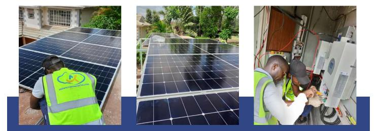
Customer: ALKINS ENTERPRISE LTD Type: Rooftop solar power plant Installed capacity: 6.6 kWp Region: JUJA KIAMBU COUNTY Solar modules: LONGI 555 W HI-MO X6 ANTI DUST Inverters: DEYE 5kw 48v, SUN-5K-SG03LP-EU, single phase Battery:20kwh MEGA TANK GL LITHIUM ION BATTERY Works performed: design, supply of equipment and materials, installation and commissioning
