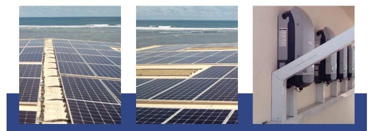
Customer: AUTOMAX ENGINEERING LTD Type: Rooftop solar power plant Installed capacity: 160kWp Region: MOGADISHU SOMALIA Solar modules: AMERI SOLAR 375 W Inverters: 25kw FRONIUS ECO 25.0-3-S, three phase Works performed: Installation
