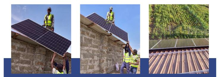
Customer: ENG KIMINGI Type: rooftop solar power plant Installed capacity: 22kWp Region: JUJA KIAMBU COUNTY Solar modules: JA Solar 575 W Bifacial Inverters: 15KW VIECHI SUNVERTER, THREE PHASE Works performed: design, supply of equipment and materials, installation and commissioning.
