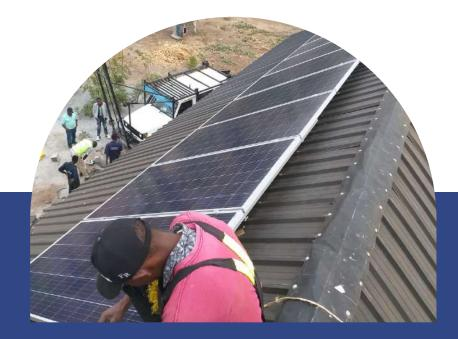
Customer: Mr. KASYOKI Type: Rooftop solar power plant Installed capacity: 6kWp Region: MWALA MACHAKOS COUNTY Solar modules: LONGI SOLAR 375 W Inverters: 4.0KW HOBBER SUNVERTER, SINGLE PHASE Works performed: design, installation and commissioning.
