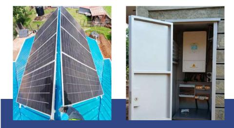
Customer: Mr. Dennis Type: rooftop solar power plant Installed capacity: 4.8 kWp Region: Kisii county Solar modules: JINKO Solar 600 W Bifacial Inverters: DEYE 5kw 48v, SUN-5K-SG03LP-EU,single phase Battery:10kwh WEKO LITHIUM ION BATTERY Year of implementation: 2024 Works performed: design, supply of equipment and materials, installation and commissioning
