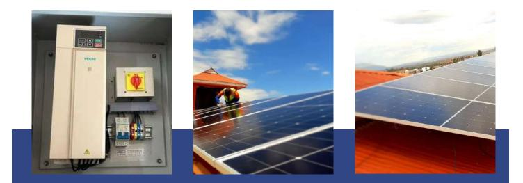
Customer: ENG KIMINGI Type: rooftop solar power plant Installed capacity: 16 kWp Region: JUJA KIAMBU COUNTY Solar modules: LONGI HI-MO X6 ANTI DUST 575 W Inverters: 11KW VIECHI SUNVERTER, THREE PHASE Works performed: design, supply of equipment and materials, installation and commissioning.
