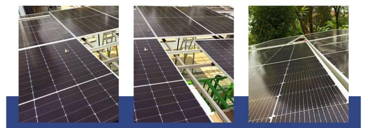
Customer: JEMIGREEN LTD Type: rooftop solar power plant Installed capacity: 6.25 kWp Region: Eldoret Uasin Gishu county Solar modules: JA Solar 575 W Bifacial Inverters: DEYE 5kw 48v, SUN-5K-SG03LP-EU,single phase Battery:10kwh U-HOME LITHIUM ION BATTERY Works performed: design, supply of equipment and materials, installation and commissioning
