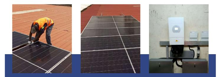
Customer: JEMIGREEN LTD Type: Carpark solar power plant Installed capacity: 10 kWp Region: Eldoret, Uasin Gishu county Solar modules: LONGI 625 W Inverters: DEYE 8kw 48v, SUN-8K-SG03LP-EU, single phase Battery:10kwh MEGA TANK GL LITHIUM ION BATTERY Works performed: design, supply of equipment and materials, installation and commissioning
